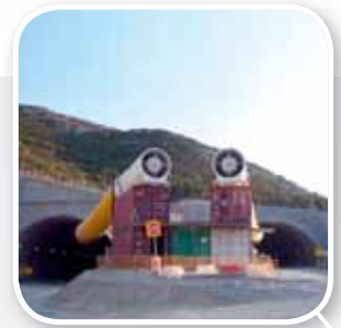
Maliakos-Kleidi road tunnel, Greece
