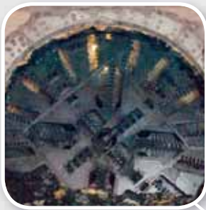
A86 Duplex tunnel, France
