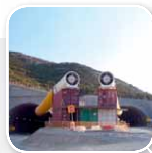
Maliakos-Kleidi road tunnel, Greece
